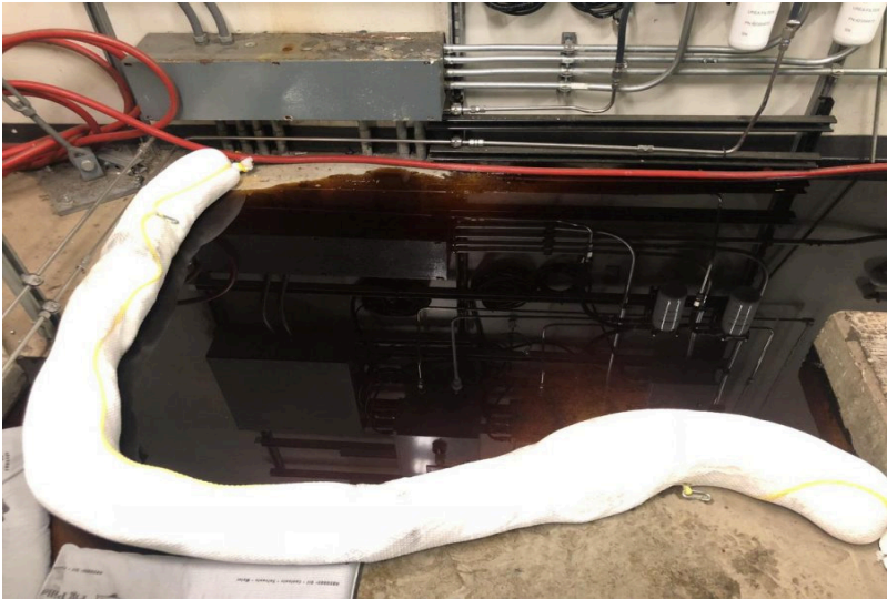
Oil spilled all over the Energy Center's floor after a generator fire.
